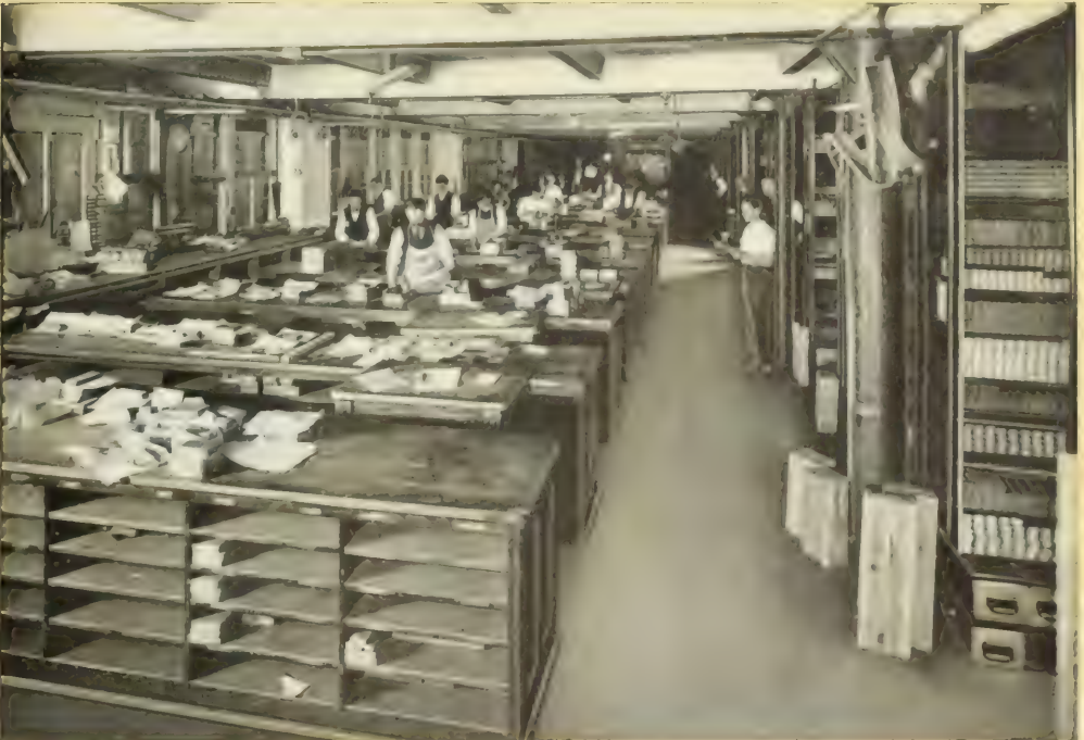
CORNER OF THE SHIPPING ROOM
